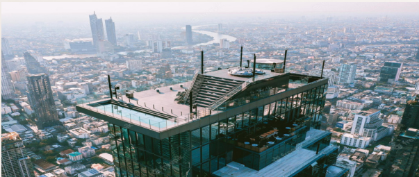
KING POWER MAHANAKHON 114 Naradhiwas Rajanagarindra Rd, Silom
